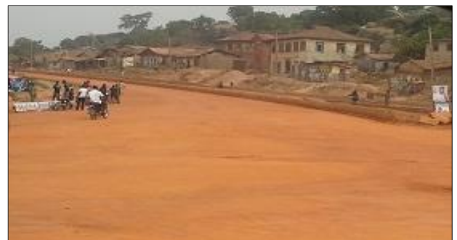
Fig 5: Ikija Road expansion in progress
